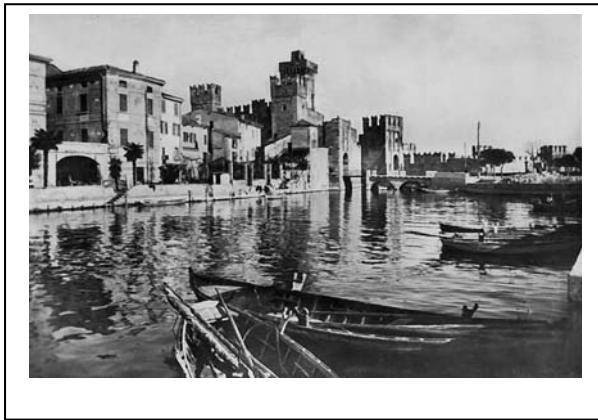
Photo M39 Date: 1940-06 Location: Lago di Garda, Italy Showing: Sirmione
